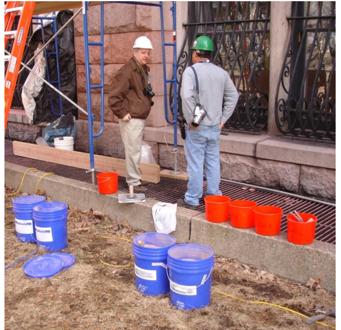
Repointing Mortar Mock-ups at AMNH, 2007
