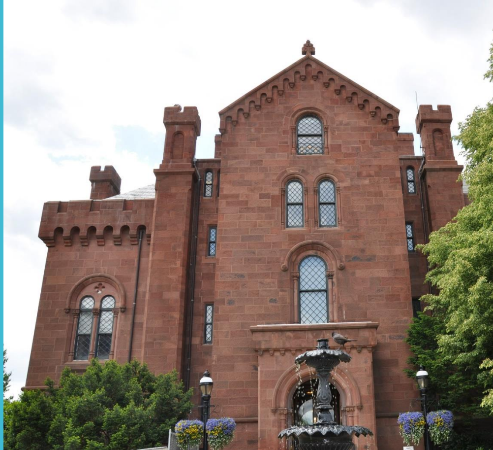
SPOT REPOINTING WITH LIME PUTTY MORTAR AT SMITHSONIAN CASTLE
