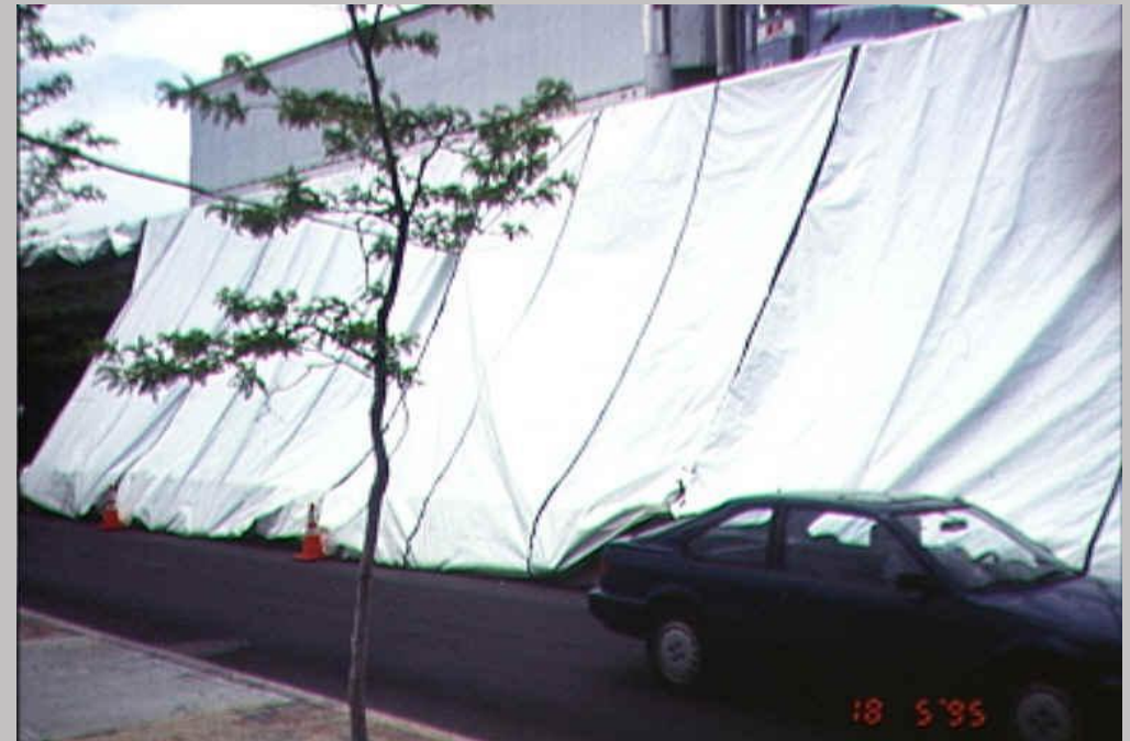
Abrasive blasting containment
