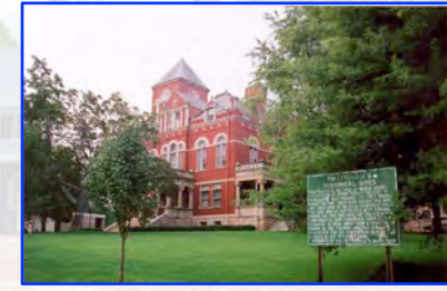
Fayette County Courthouse, Fayetteville, WV Lime-pozzolan, hydraulic lime mortar
