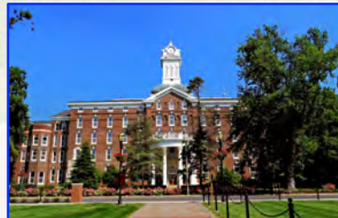
Kutztown University, PA 1880s hydraulic lime mortar
