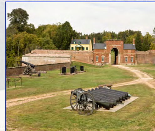
Fort Washington (Maryland) Hydraulic lime mortar, circa early 1800s
