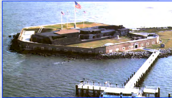
Fort Sumter (Charleston, SC) Natural cement concrete Natural cement – lime mortar, circa 1850
