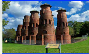
Saylor Park Cement Kilns, Coplay, PA 1890s early Portland cement- lime mortar
