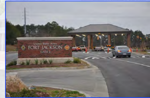
Fort Jackson (Columbia, SC) Masonry cement pointing mortar, circa 2009
