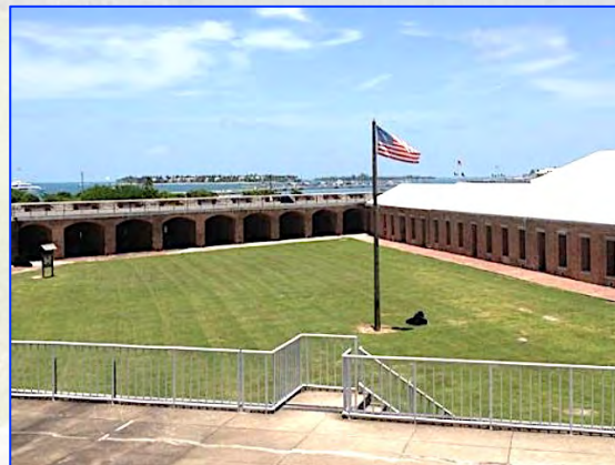
Fort Zachary Taylor East (Key West, FL) Natural cement – lime - beach sand mortar, circa 1845
