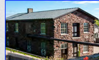
Canal Stores Building, Sault Ste. Marie Canal, Canada 1895s lime mortar
