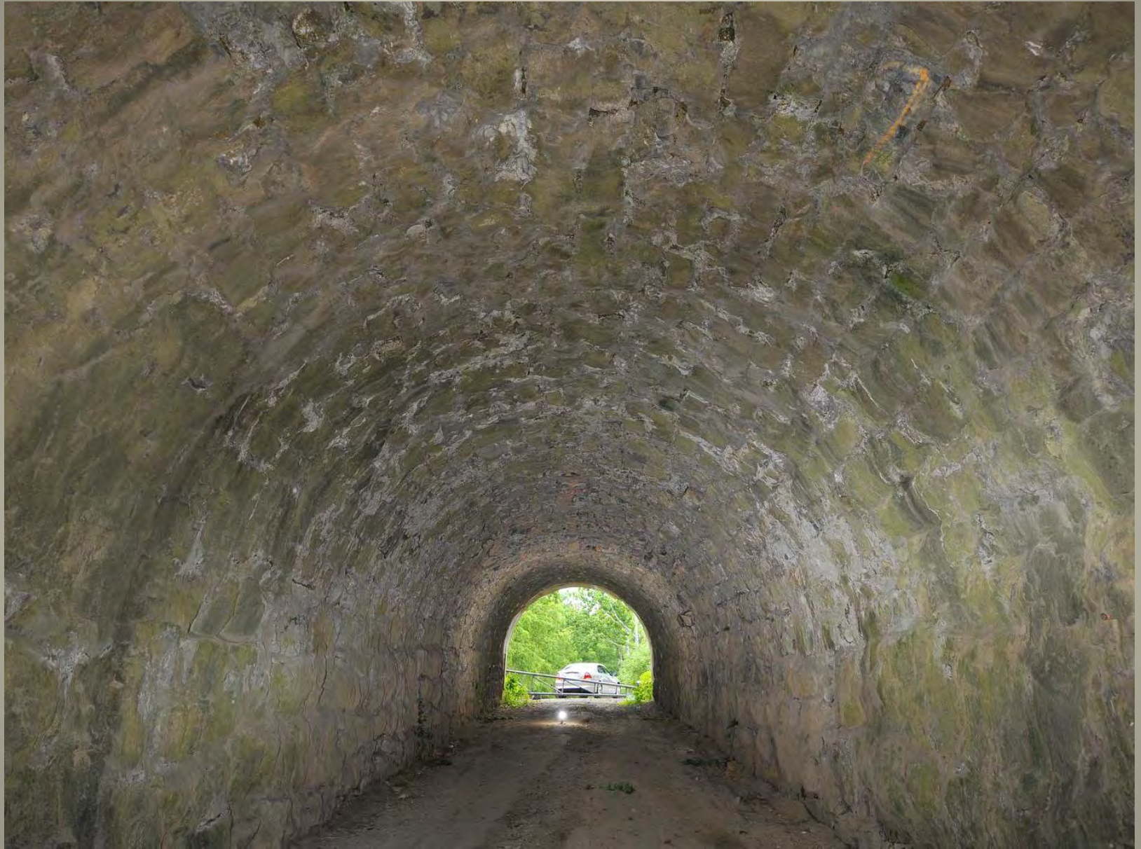
Still Valley Railroad Tunnel
