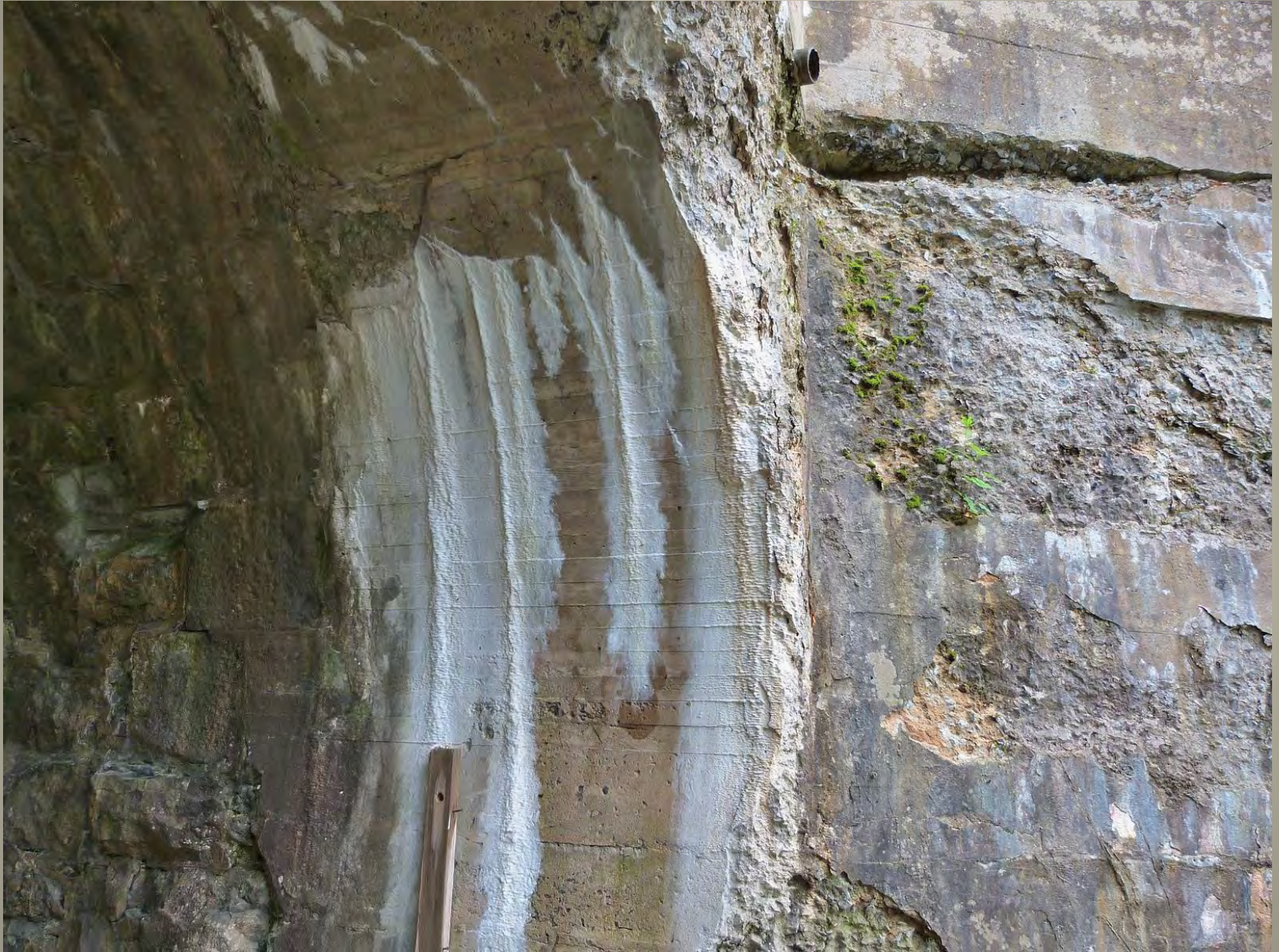
Still Valley Railroad Tunnel
