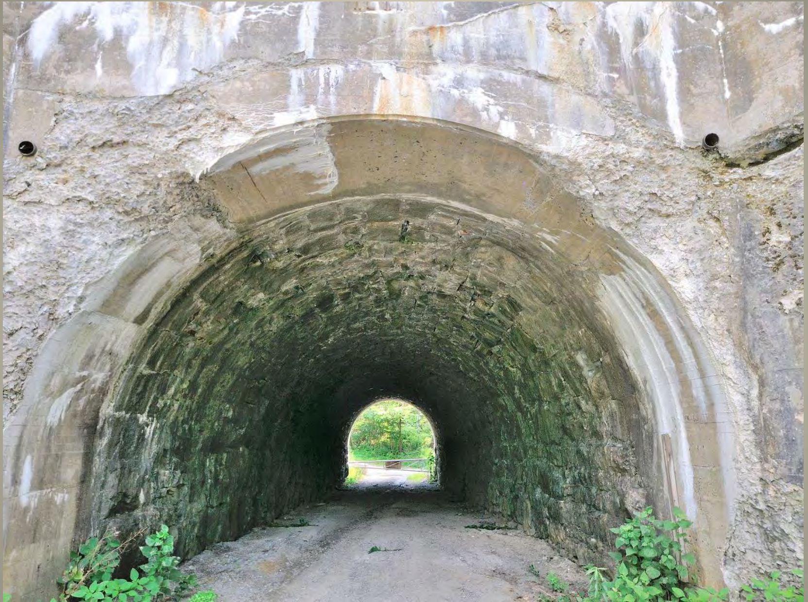
Still Valley Railroad Tunnel
