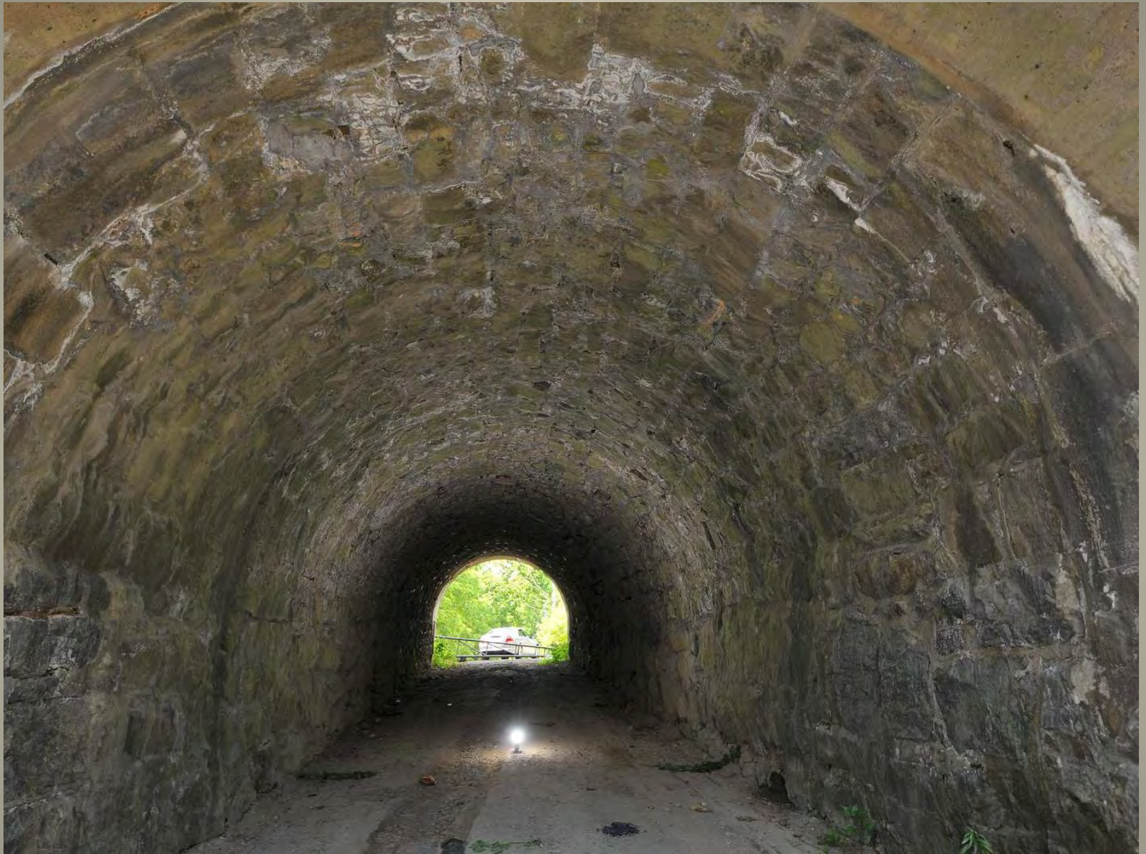
Still Valley Railroad Tunnel
