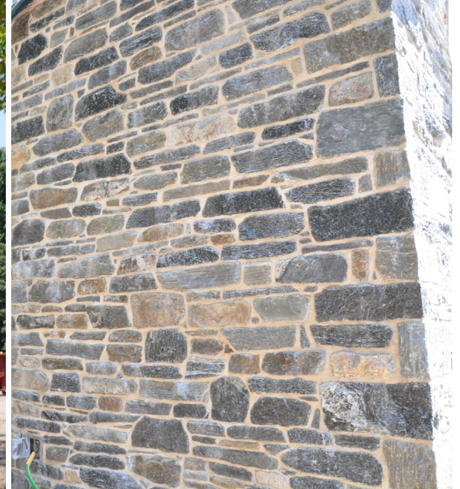
RESTORED 2008, LIME-SAND MORTAR CHIMNEYS REBUILT W/TYPE K MORTAR
