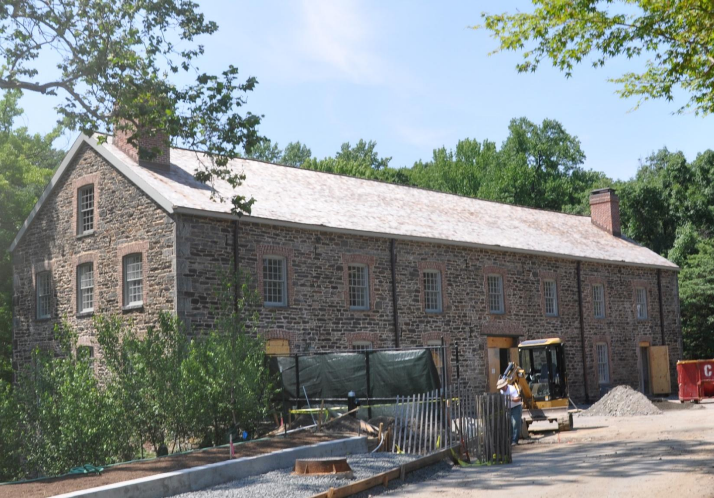
NY BOTANIC GARDENS STONE MILL BUILT 1840, LIME-SAND MORTAR
